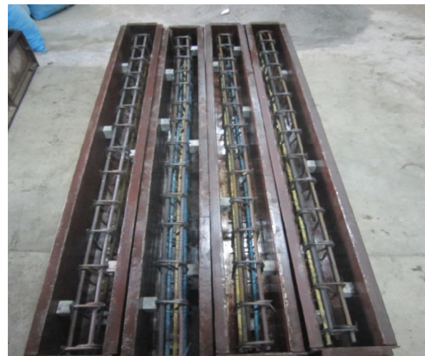
Figure 3.2 Arrangement of cover with reinforcement
