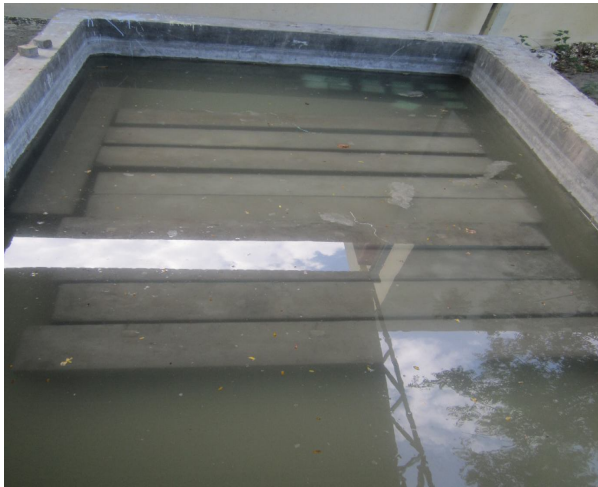
Figure 3.4- Beams at the time of curing
