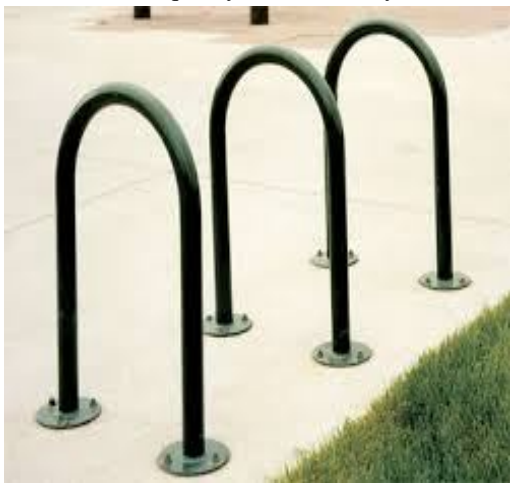
Figure 1: - Rack design (U-rack)
