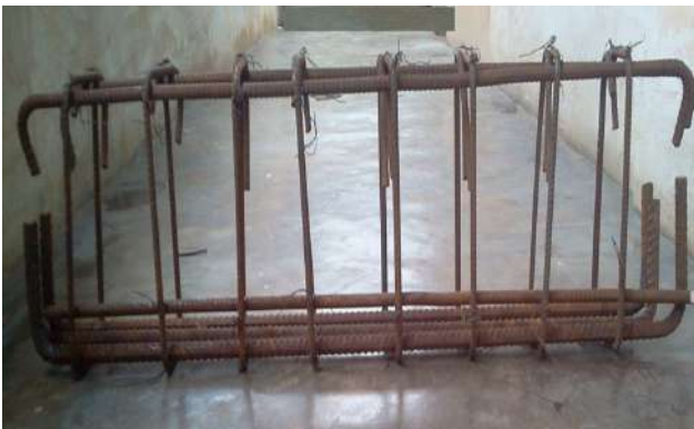
Figure 15. Reinforcement of ORB
