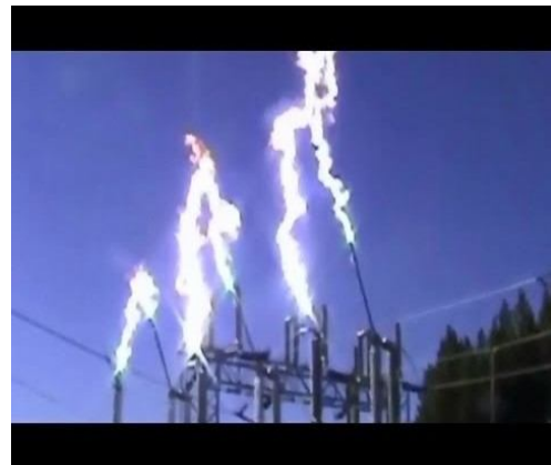
Figure 11 arc production in isolator
