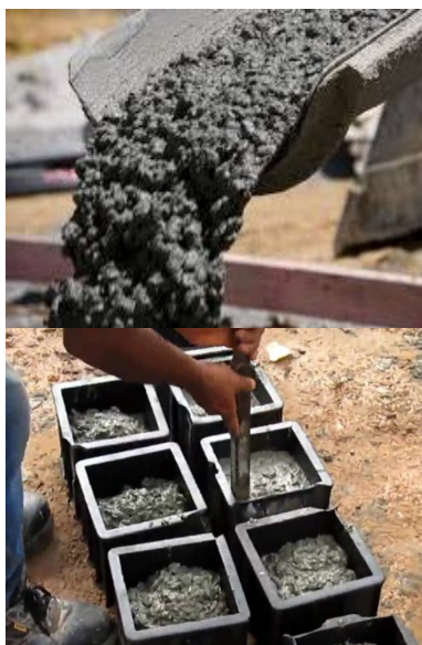
Fig1.1: laying of concrete
