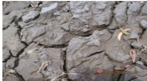
Fig 2.3 Cracks in Marine Clay Deposits
