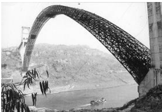
Fig.6 Arch rib being erected
