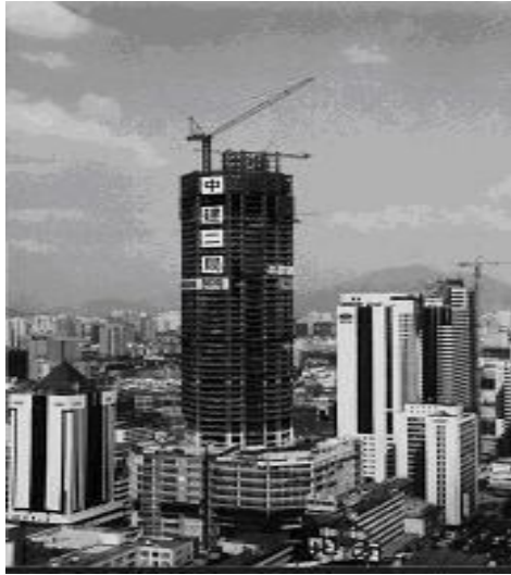
Fig.7 SEG Plaza under construction
