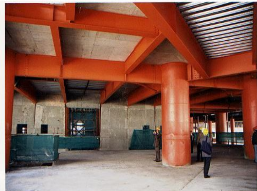
Fig. no.4 Composite steel story system
