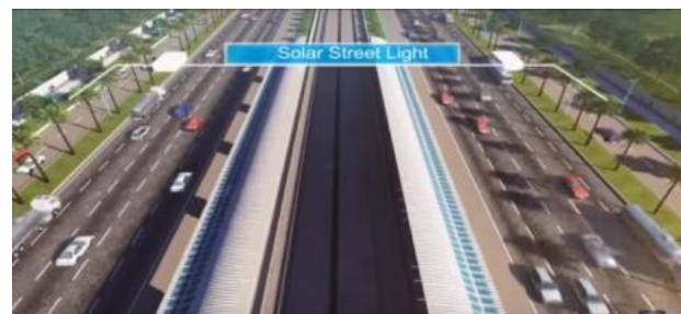
Fig 3.4: metro with solar street light
