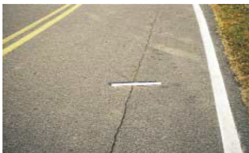
Plate 2.3 Failure Crack
