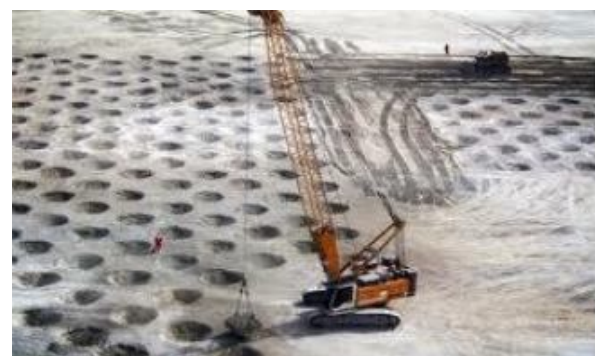
Fig.5 dynamic compaction
