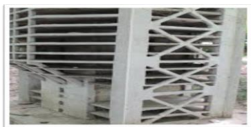
Fig. 1 Provision diagonal bracing
