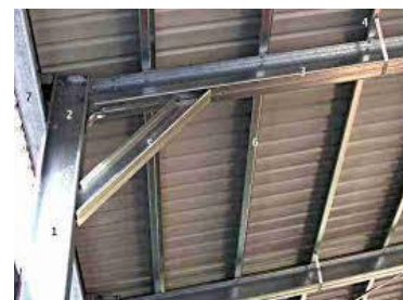
Fig.3 Knee bracing
