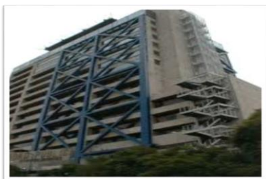
Fig.2 Retrofitting by diagonal bracing
