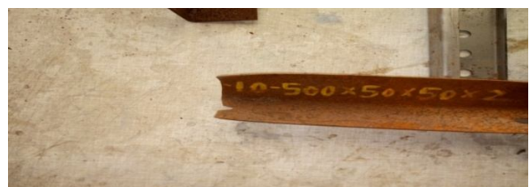
Fig 9 Failures due to block shear of single unequal angle specimen 50x50x2
