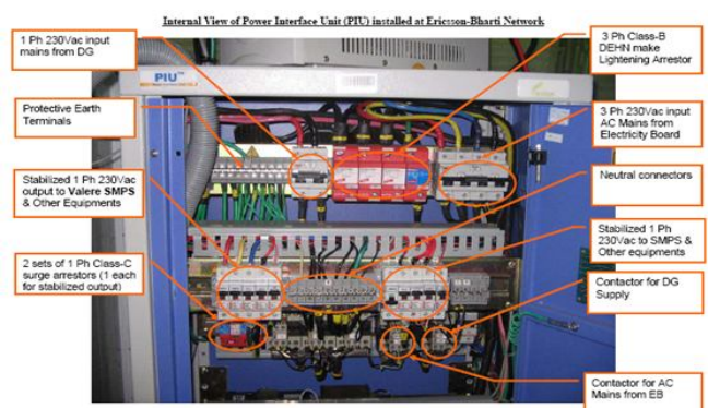
Fig.3) Example of Power Interface Unit (PIU)
