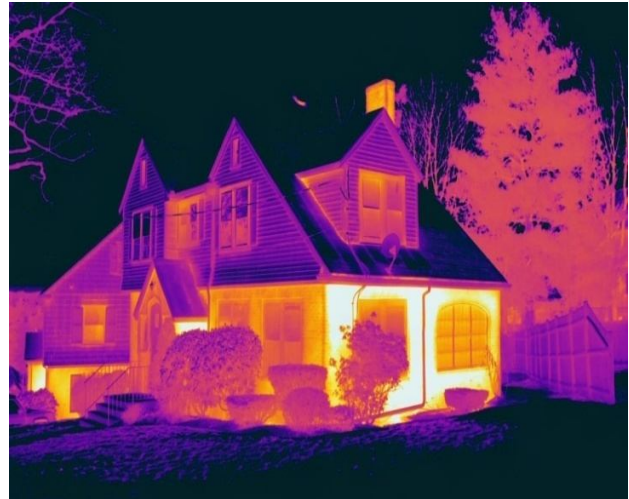
Fig4: captured image by thermal imaging system
