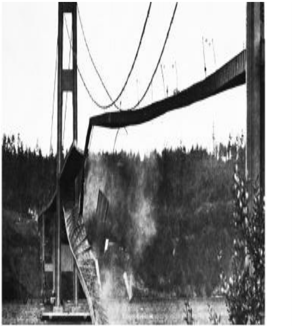
Fig.1 Tacoma narrow bridge during wind induced vibration. The bridge open on July 1 1940 and collapsed on November 7 1940
