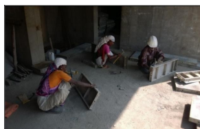
Cleaning of formwork
