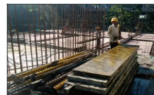
Oiling of formwork
