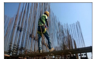
Fixing of bars
