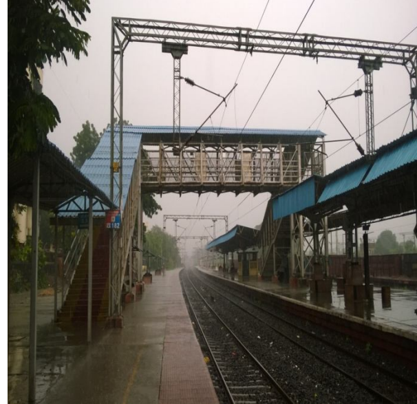
Fig.:- Foot Over Bridge
