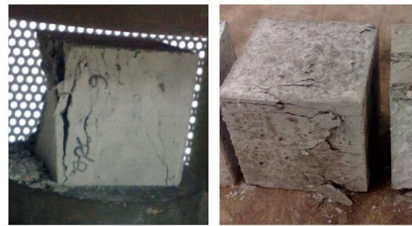
Figure 4. Samples shape after failure
