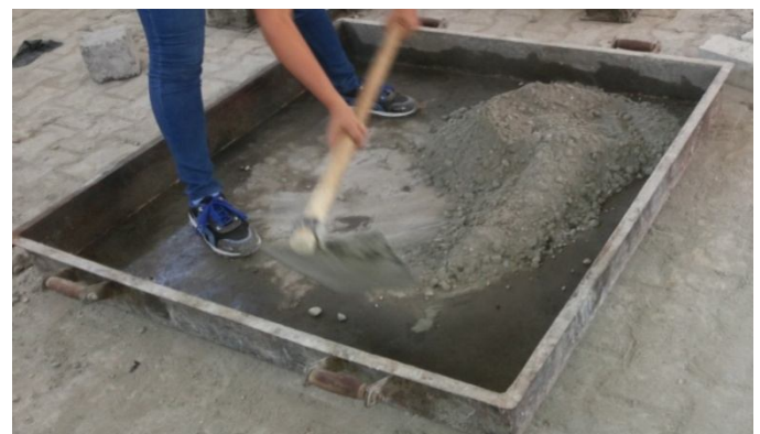
Fig. Mixing of concrete
