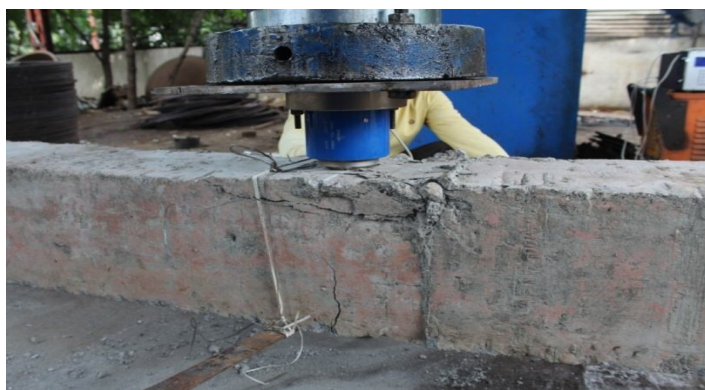
Photo No. 3.4: First crack at centre of beam.
