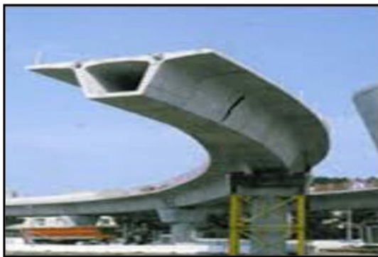
Fig:-1 Pres-stressed Concrete Trapezoidal Box Girder Bridges.
