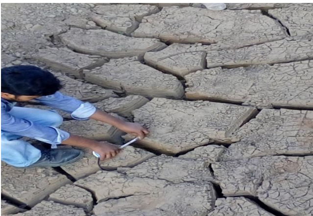
Figure 2. Expansive Soil Showing Cracks
