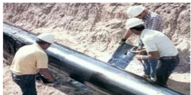
FIG. 2.1: Coating Newly Installed Pipe for Corrosion Control
