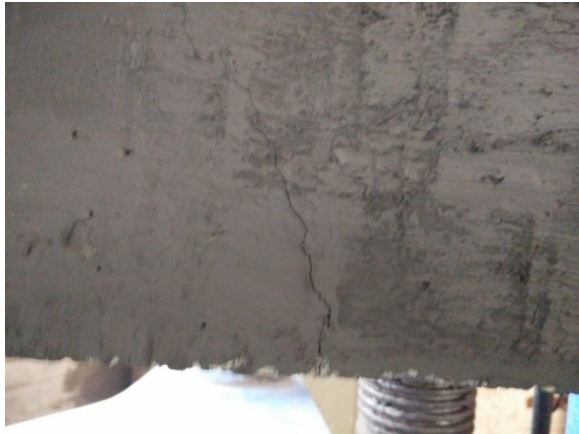
Figure 8. Crack on surface of B2
