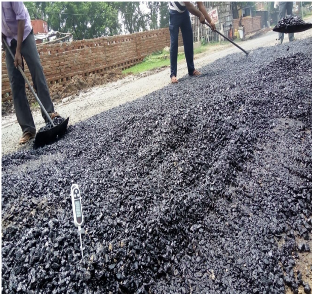
Fig 7.1 – Thermometer used for temperature measuring in bituminous
