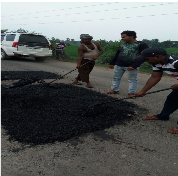
Fig 7.2 – Upsetting of bituminous
