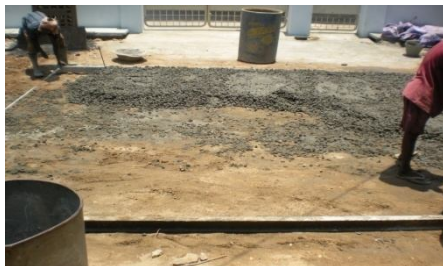
Fig. 5.2 Placing of Forms
