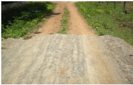
Fig. 5.1 Preparation of Subgrade Soil & Sub-base
