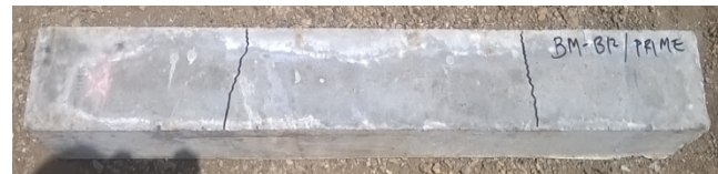
Figure-18. Crack pattern of the failed specimen BM-B12-415
