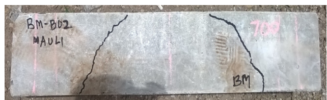
Figure-15. Crack pattern of the failed specimen BM-B02-1-500
