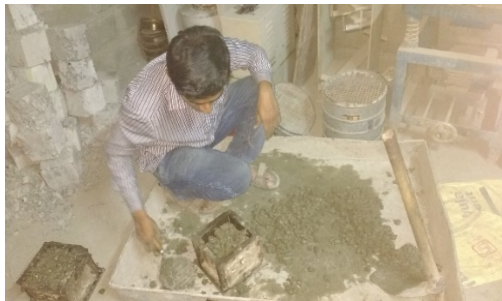
Figure 2 Mixing of materials
