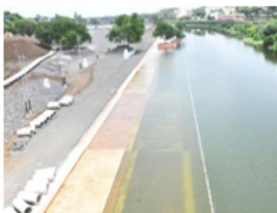
3)laxminarayan bridge – 8000sqm
