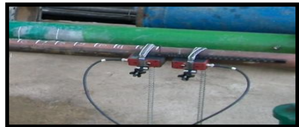
Fig. 2: Installation of ultrasonic flow sensors at straight pipe
