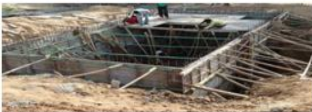
Fig 1 : Construction of Underground Tank
