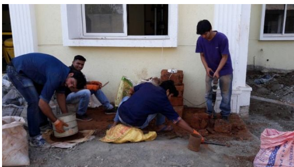
Breaking & sieving of Scrap laterite blocks to make aggregates
