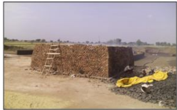
Fig. 4 Kiln for baking bricks
