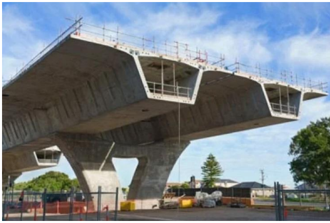
Fig 1: Precast Segmental Bridge
