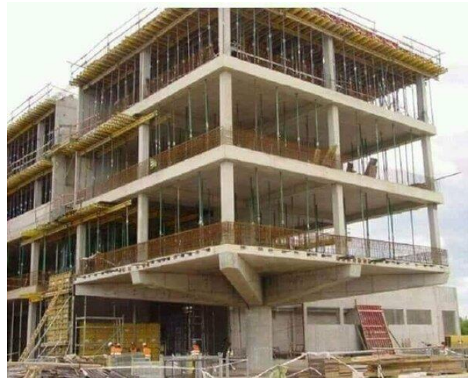
Fig 1: Floating column used on Structure in construction
