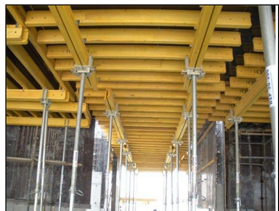
Fig. no. 1 Shuttering of flat slab
