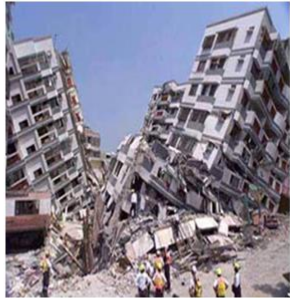
Fig 1.1: Collapse of building due to earthquake
