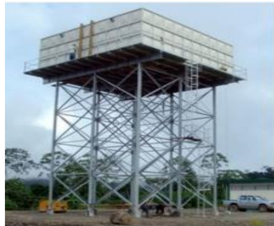
Fig 1: Elevated water storage tanks (ESR)
