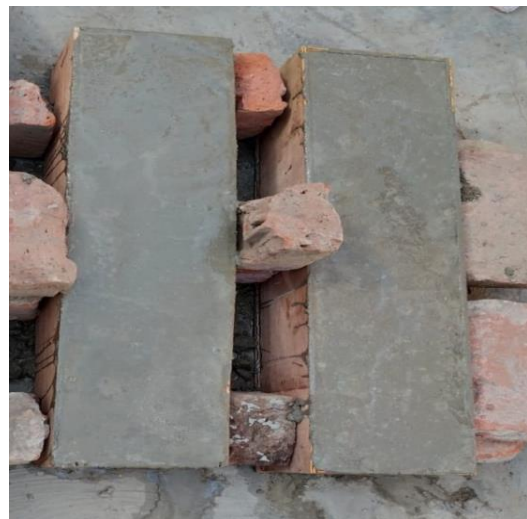
Figure 3. Casting of beam
