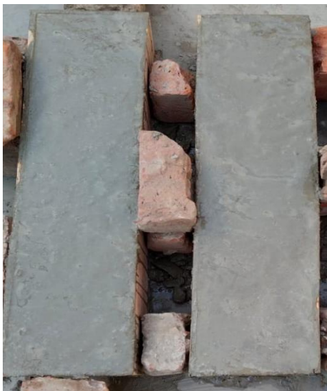
Figure 5. Casting of beam
