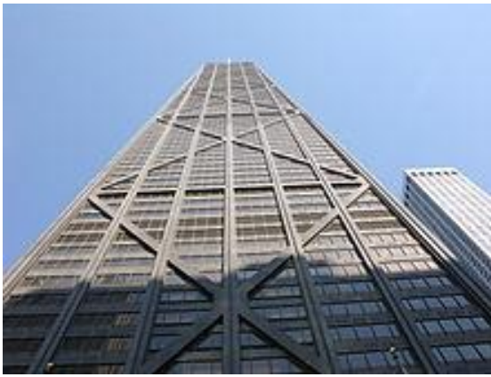
Fig 3. 1:Cross bracing
