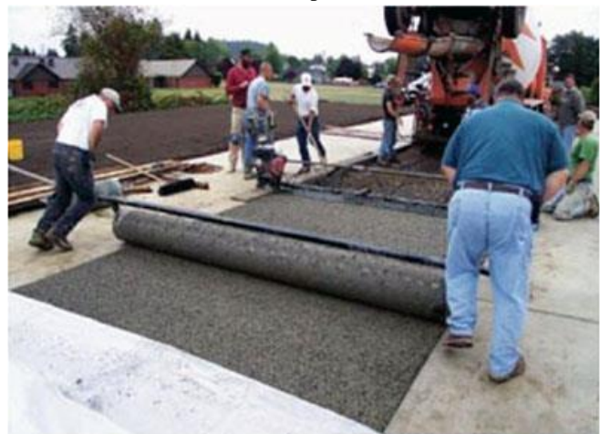
Fig 5.1 Placement And Consolidation
