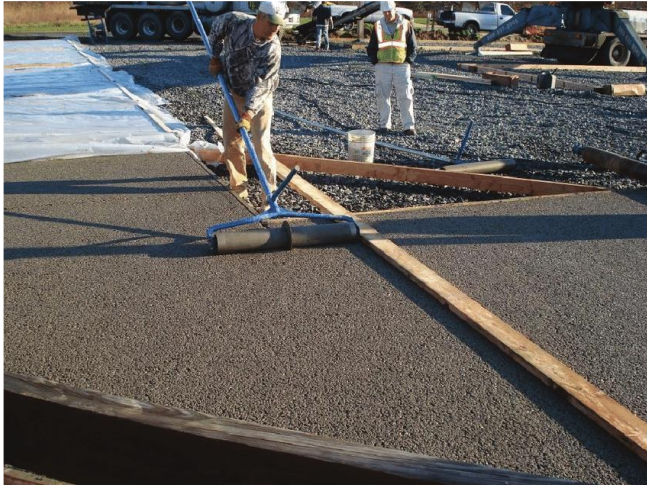
Fig 5.2 Joint Placement
