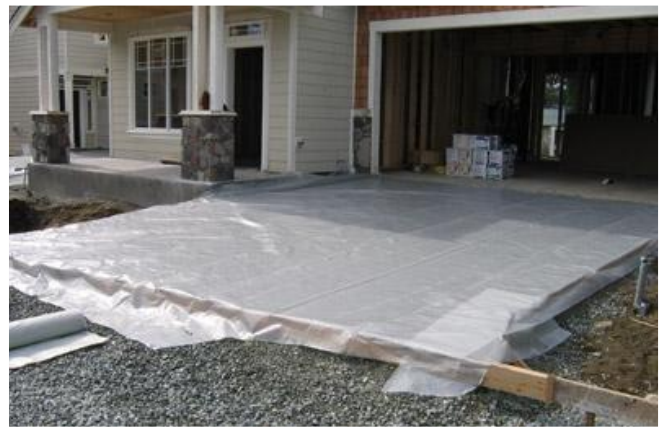
Fig 5.3 CURING AND PROTECTION
