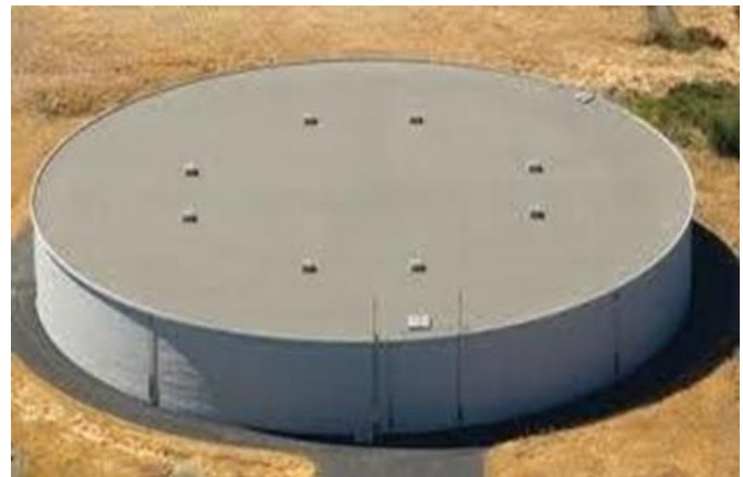
Fig No 1: . Tanks Resting On Ground
