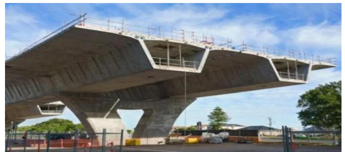
Fig 1: Precast Segmental Bridge
