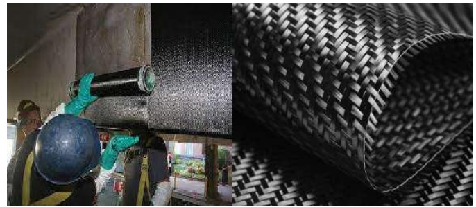
Figure 5: CFRP Sheet Wrapping Technique
