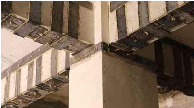
Figure 6: External Plate Bonding Method
