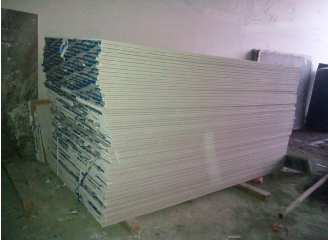
Photo no 1: storing of gypsum boards
