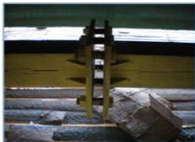
Pre-stressing Mechanism in Truss
