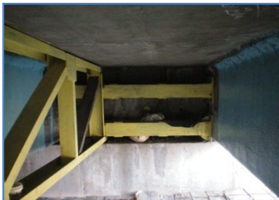
Connection of truss over main beam
