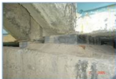
Replacement of damaged Bearings
