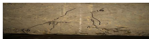
Appearance of beam after testing
