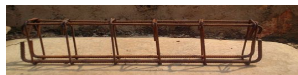
Reinforcement of CSB
