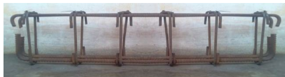
Reinforcement of OSB
