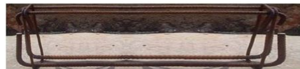
Reinforcement of stirrups at the end of beam
