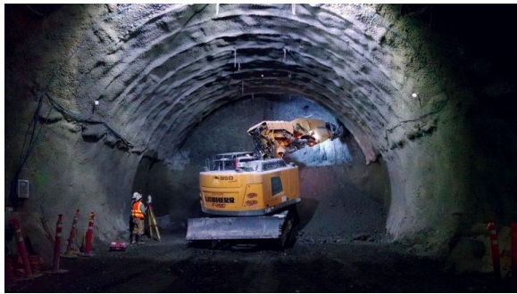
Fig NATM Drilling process
