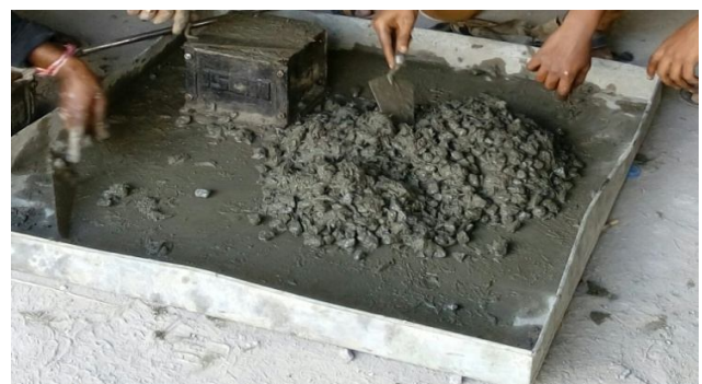
Figure 2: Mixing Of Concrete
