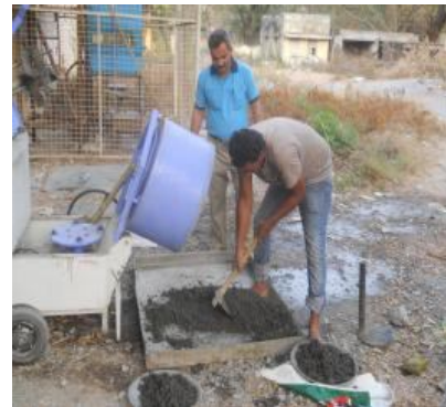
Figure 2. Wet material mixing(C)
