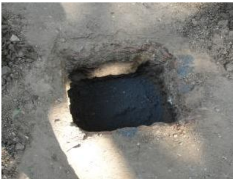
Figure 4. A View of Pit for Construction of Test Section
